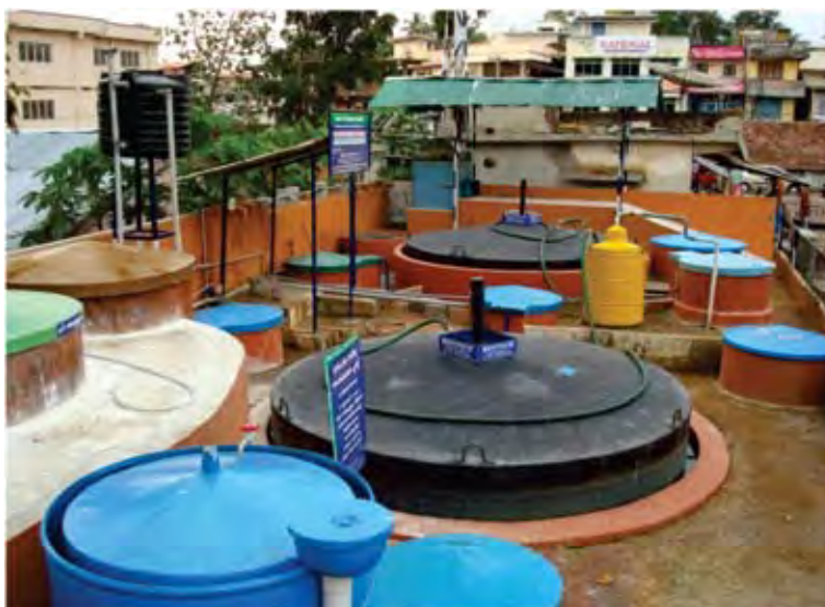
Waste to electricity plant
